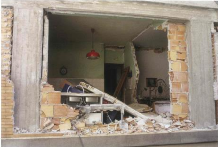
Fig. 4.1: Collapse of non-structural components in a residential building, 2009 Abruzzo Earthquake, L'Aquila, Italy
